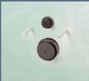
The protective plugs are simply pushed onto the flush pipe and drain bend.
