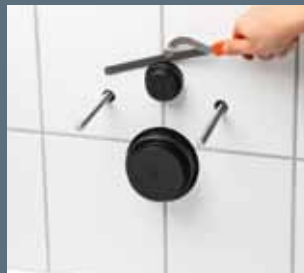
The protective plugs can now be cut flush to the surface with a saw blade.
