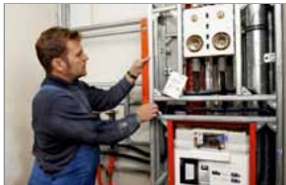
... Installation of the prefabricated modules on the construction site ...
